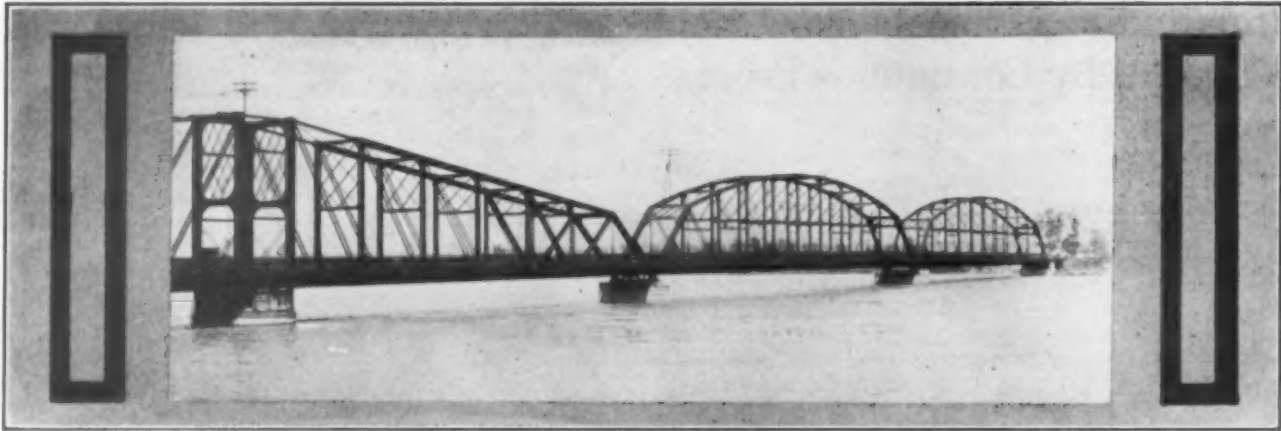
The Chicago Great Western Bridge Over the Missouri River at Leavenworth, Kan.
